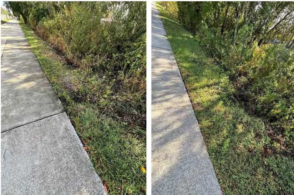
**Location 2:** Overgrown vegetation needs to be cleared and bank needs to be regraded to original condition. The slope should be stabilized with flexamat from the existing sidewalk to the toe of slope of the existing ditch. Sod all disturbed areas and replace all broken concrete as needed due to the repair.
