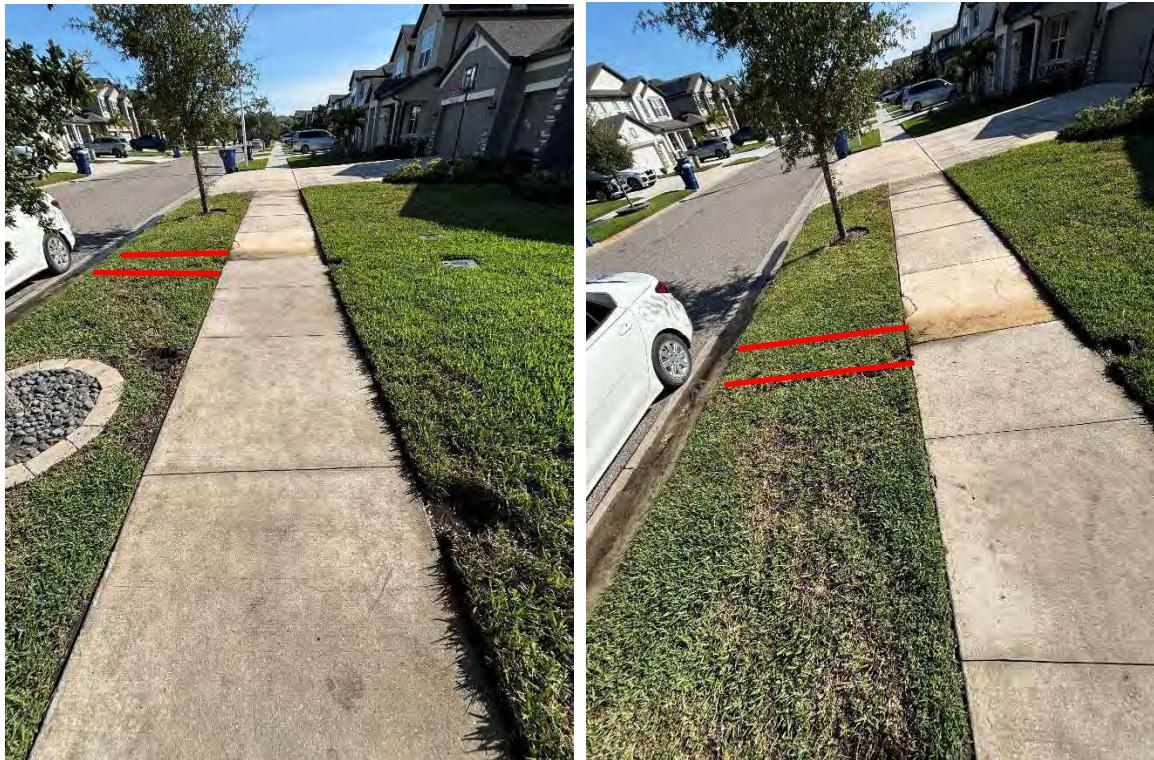
**Location 2:** Install a flume at the low point of the sidewalk to divert water from sidewalk to the curb.
